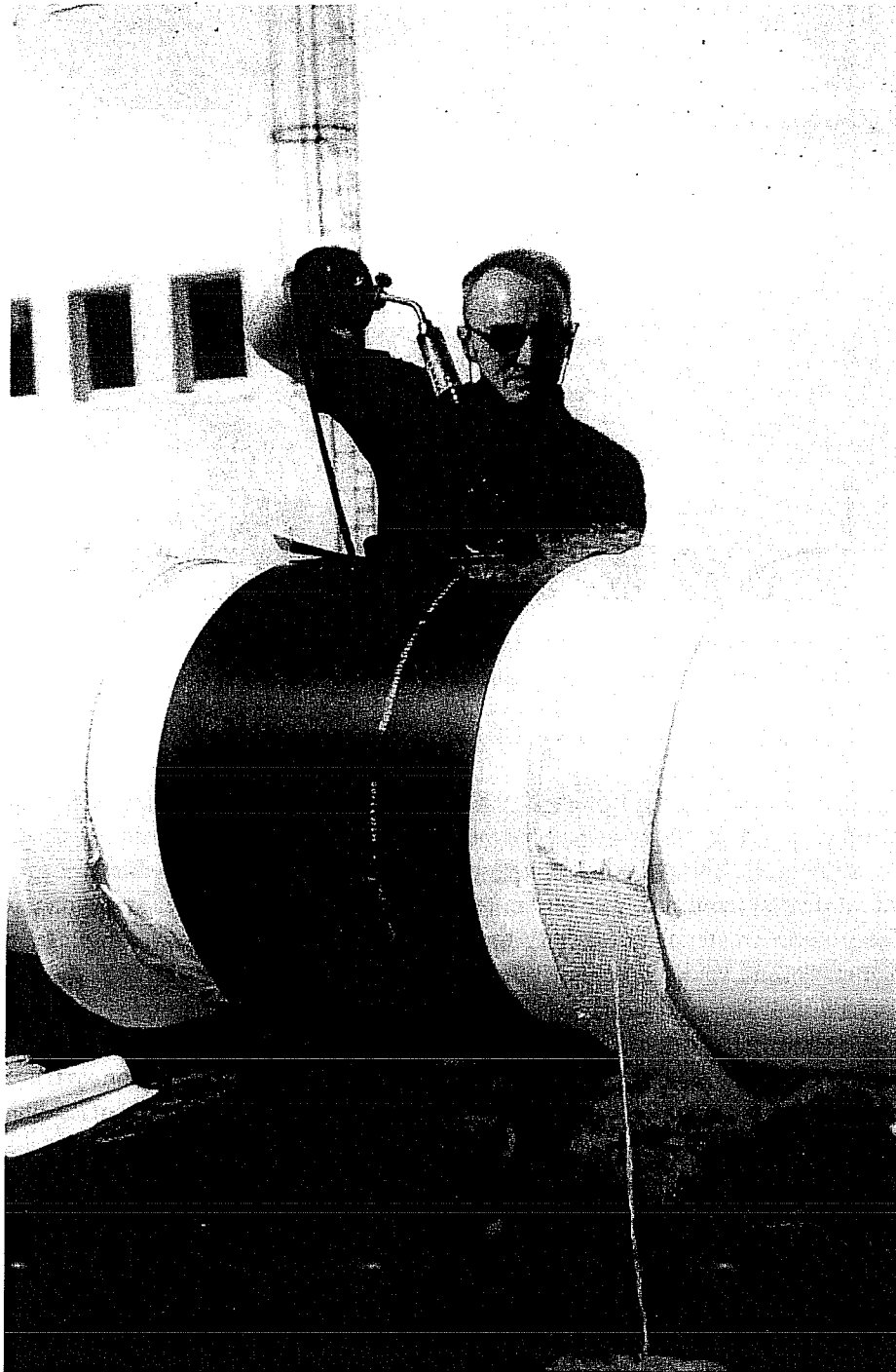
FIGURE 18.29 On-site corrosion protection of the welding area — shrinking method. (Courtesy of Siemens.)
