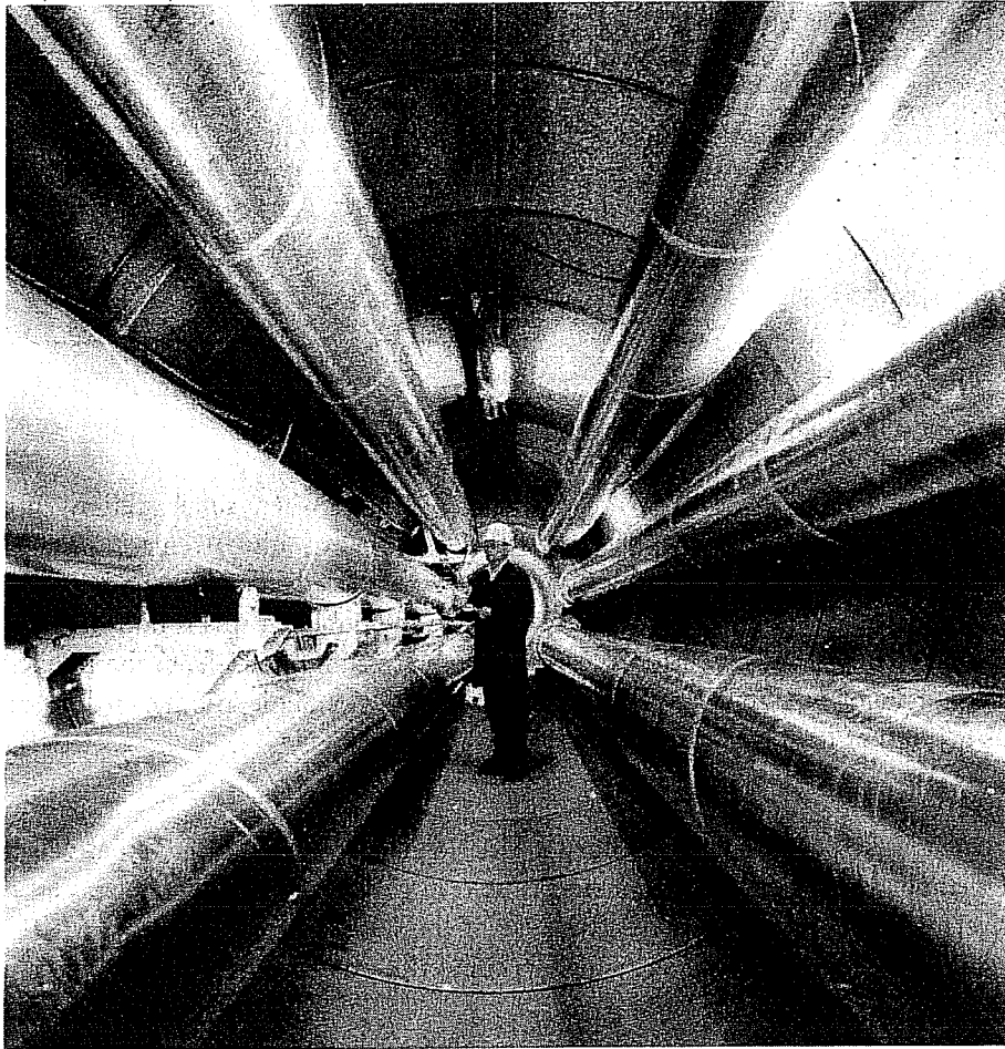
FIGURE 18.7 View into the tunnel. (Courtesy of Siemens.)
