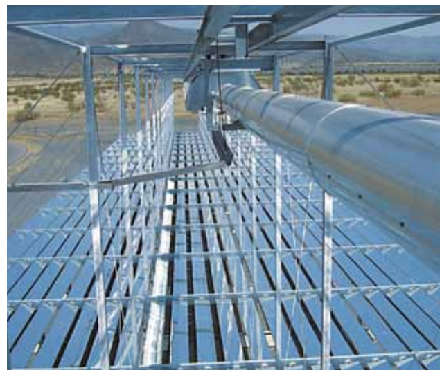
Figure B.7 – Linear Fresnel concentrator plant
